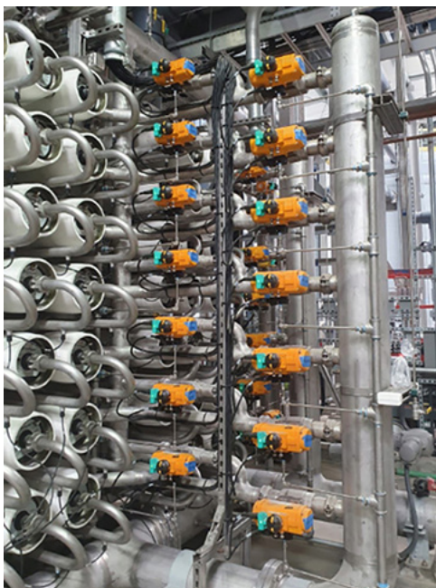
Valves (orange) installed on existing RO during ROTEC FR-RO retrofit
