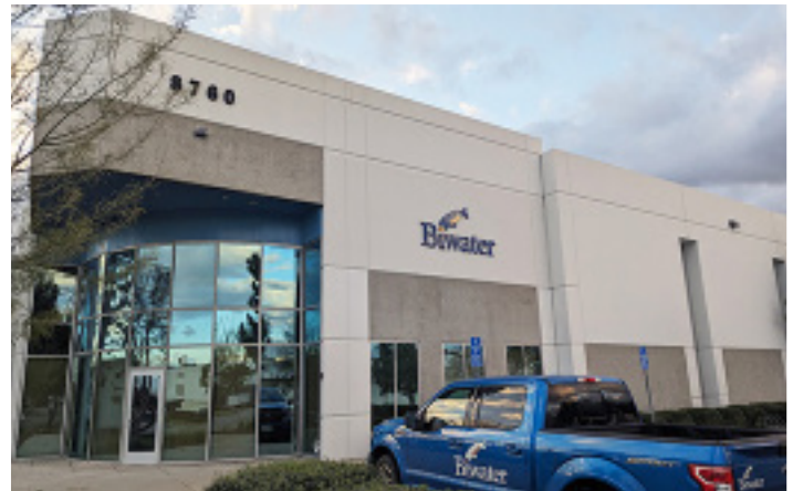
Biwater's new Cucamonga facilities, east of Los Angeles
